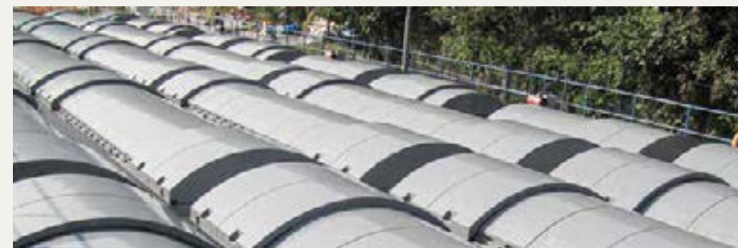
Project Owner: Water Suppliers Department Of HKSAR Details: Construction Of FRP Covers To Accelerators, Settled Water Channel And Filter Bed At Shatin Water
