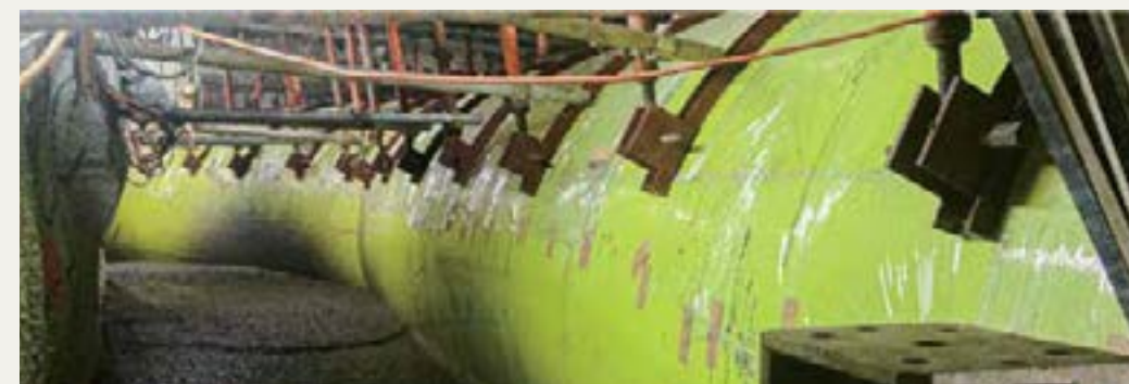
Project Owner: Drainage Serices Department Of HKSAR Details: Provision Of FRP Formworks To The Concreting Of Sewage Conveyance System From North Point To Stonecutters Island. Across Victoria Harbour
