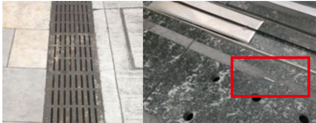
7. Material spalling off due to internal rusting
